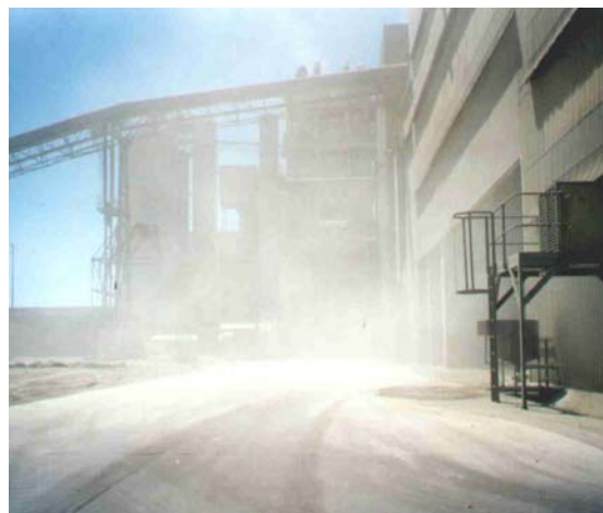
Figure 7: The cement dust laden environment of Whites North Substation
